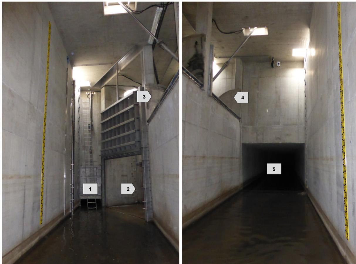
Figure 1-2: Sluice gates to WWTP Graz [1] and to the river Mur via the overflow channel [2] and moveable weirs to the overflow channel [3], [4]; storage volume upstream of CS 1 [5] (images: Graz University of Technology, 2014)
