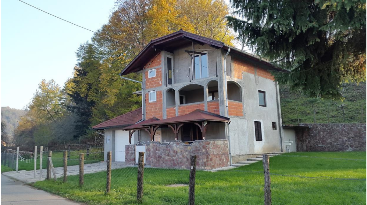
Figure 44: The mismatched use of the materials and semi-circular openings; view from the south-west
