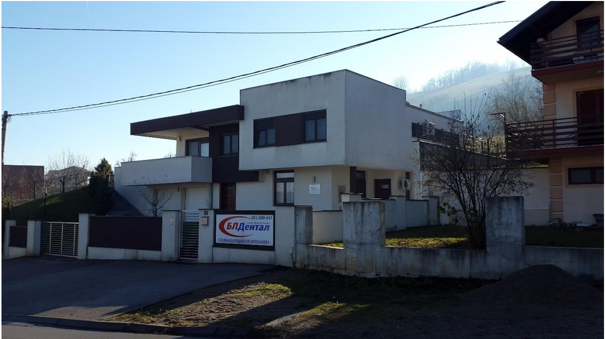
Figure 51: Contemporary house on the city hill with dental clinic; view from the south-west
