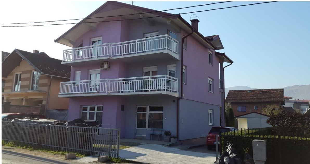
Figure 27: Different colours on the façade for accentuating the house geometry, view from the north-western corner
