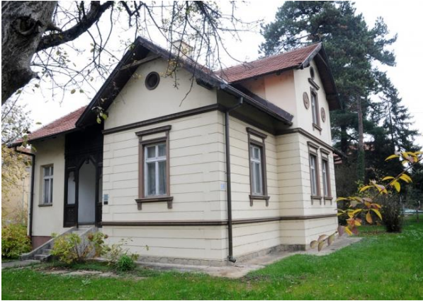
Figure 8: House of Vlado Milosevic; view from the south-eastern corner; present condition
