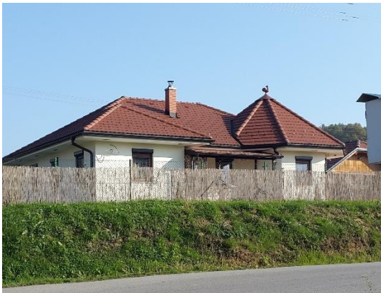
Figure 36: Geometric addition on a ground floor house corner; view from the west
