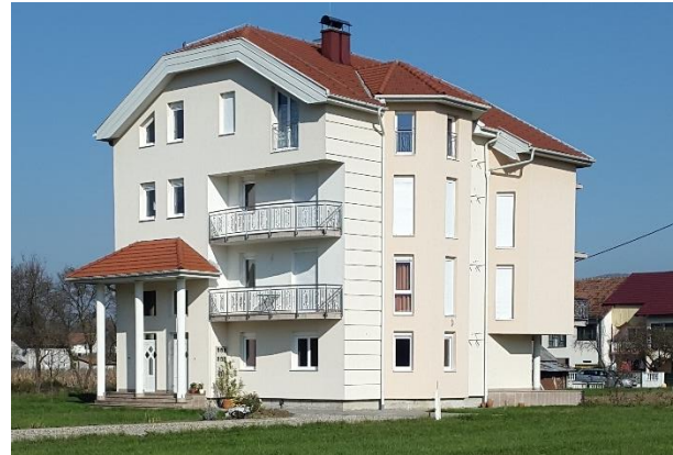
Figure 37: Geometric addition in the middle of a four storey house; view from the south-eastern corner
