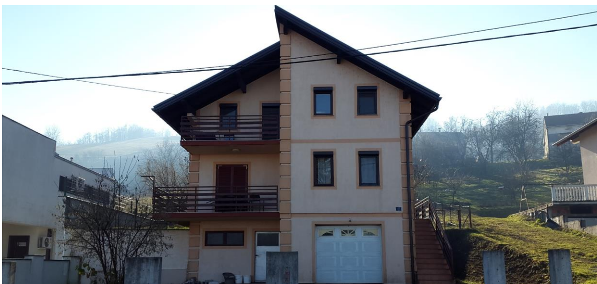
Figure 24: Emphasized corners, windows and floor division on the façade, view from the North
