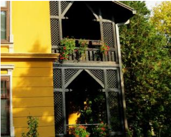
Figure 9: General Wilhelm Stockmann's villa, detail of the balcony; present condition
