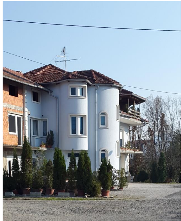
Figure 41: Excessive geometric additions, different window forms, rectangular balconies and the colour create a turbo façade; view from south
