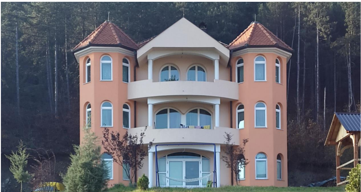
Figure 38: Two towers added on corners of a house; view from the north
