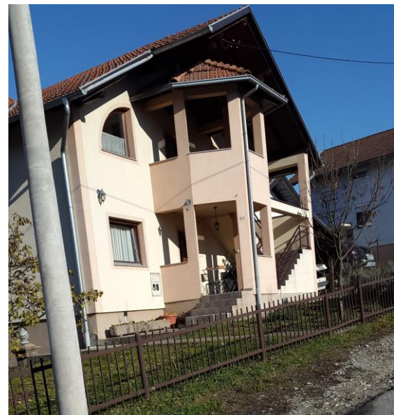
Figure 43: \frac{1}{4} circular windows, the roof and a \frac{1}{2} of an octagon added to the entrance; view from the south
