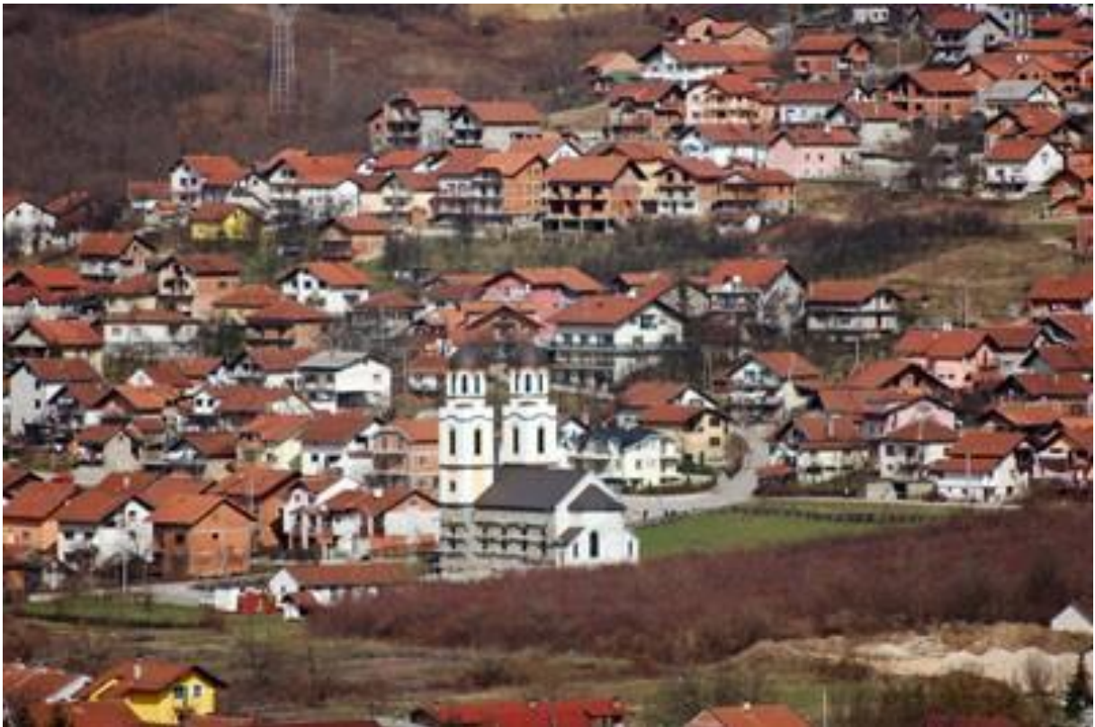
Figure 23: Settlement of Banja Luka with high number of illegally built houses
