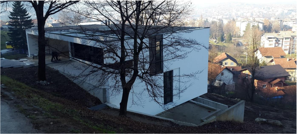
Figure 54: Recently built contemporary house, adapted to the slope of the terrain; view from the north-east
