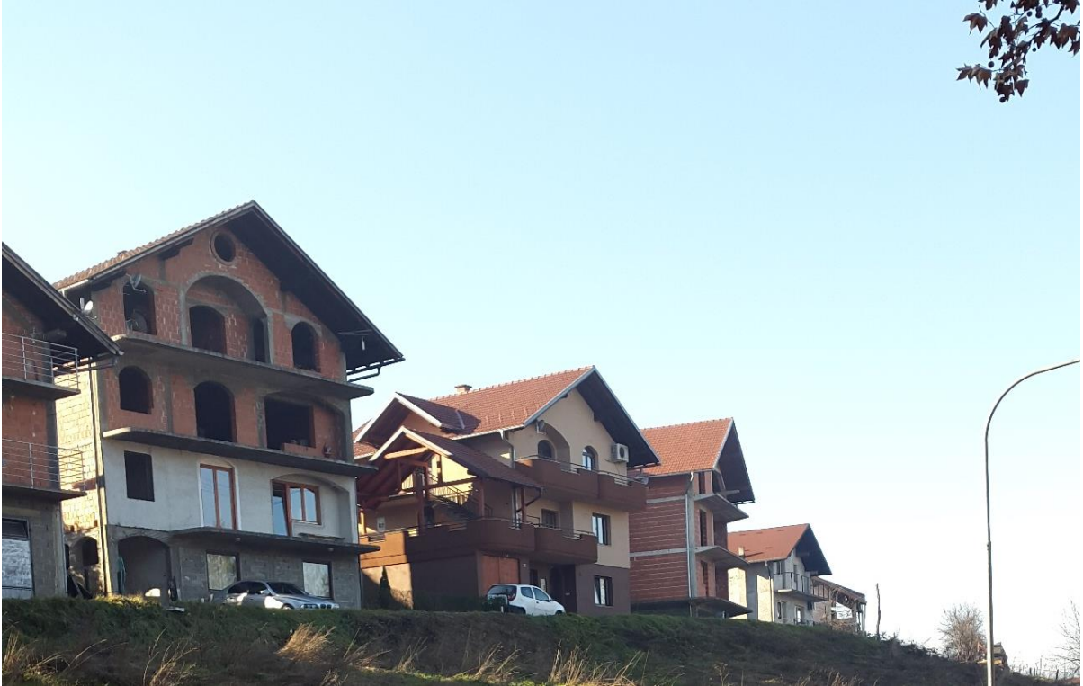
Figure 19: Line of houses in Banja Luka where only one out of five is finished
