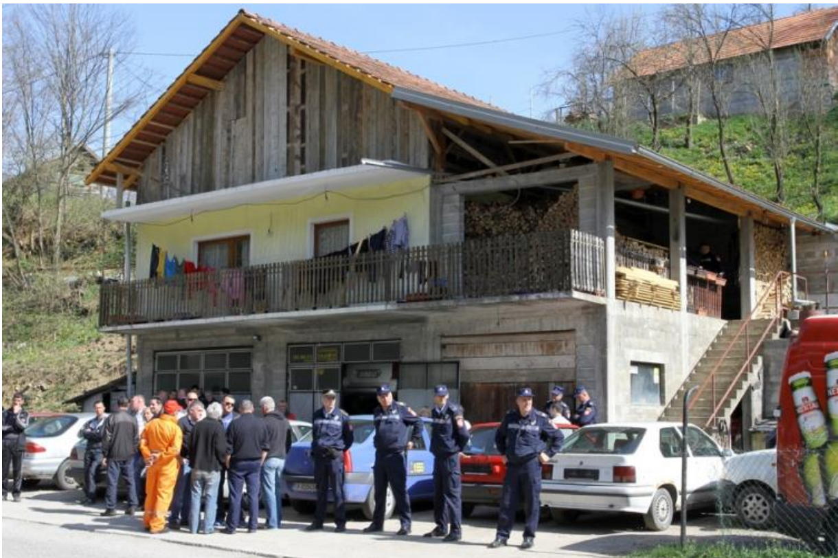
Figure 50 : Preparation for demolition of illegally built house
