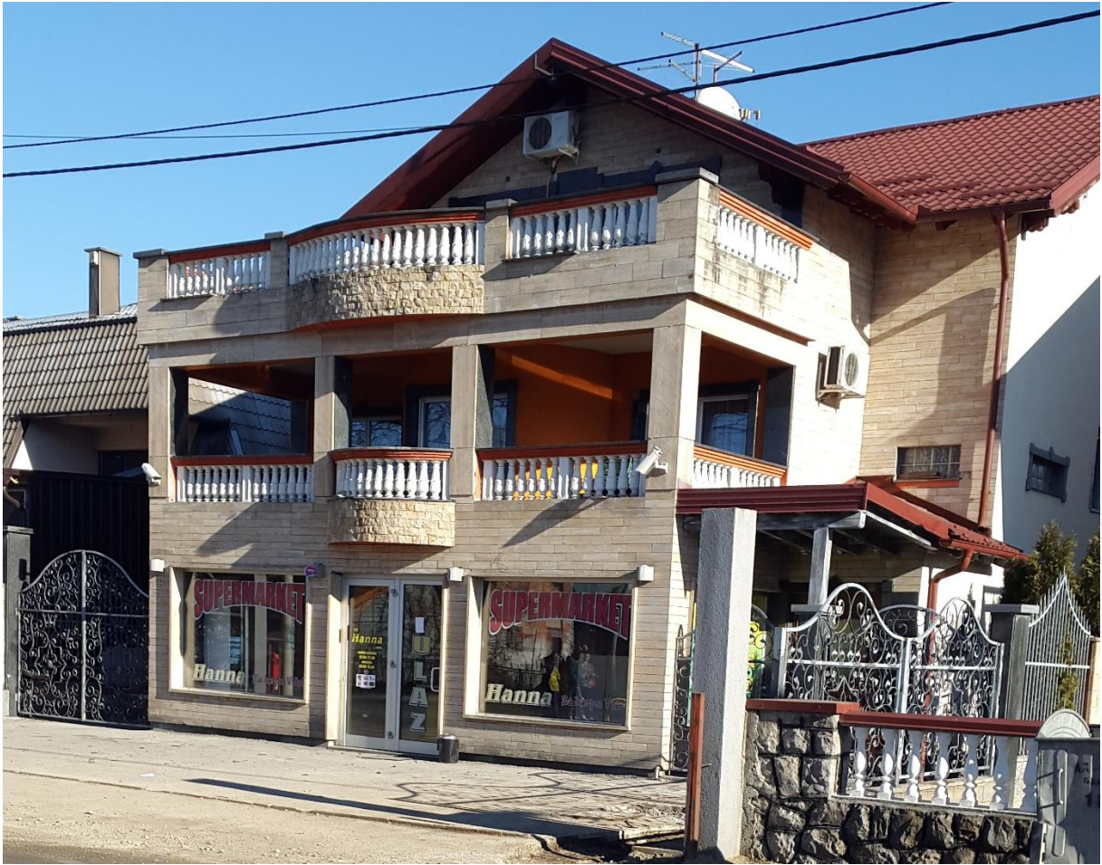
Figure 45: A turbo house with a grocery store in the ground floor; view from the south-eastern side
