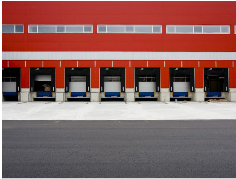
Figure 14: Eroski logistic centre automatic unloading area [23]
