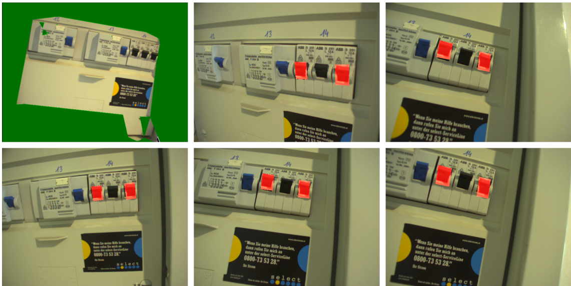
Figure 5.18: The first picture of this figure shows the created 3D model of a fuse box without applied control elements. The remaining pictures show the object and the added control elements from different camera angles.
