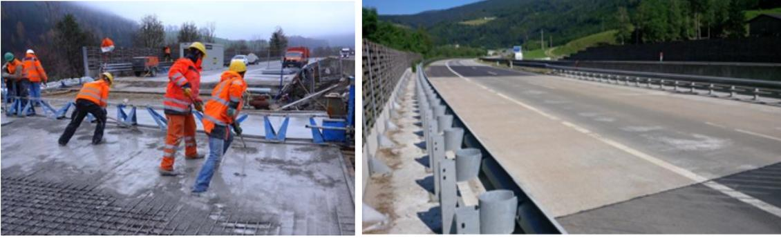
FIGURE 1.2.: Application of UHPFRC as road bridge topping within the adaptation of an existing conventional bridge to an integral abutment bridge - Steinbach bridge S6 motorway in Austria: casting the UHPFRC bridge deck (left) and the finished bridge topping (right), after Tue et al. [2015]
