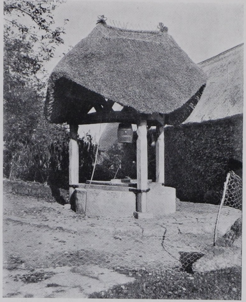
NETHERTON, SOUTH DEVON. THE RAINWATER WELL
