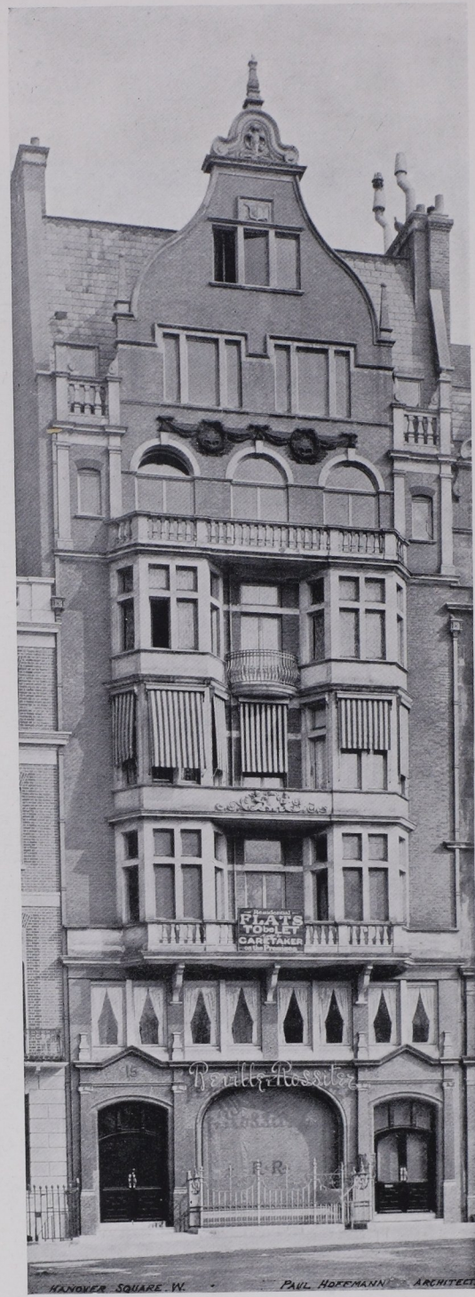
15, HANOVER SQUARE, LONDON, W. THE ELEVATION IS CARRIED OUT IN RED LEICESTERSHIRE BRICKS WITH BAYS AND DRESSINGS OF PORTLAND STONE. THE GROUND FLOOR AND THE MEZZANINE ARE IN LABRADOR GRANITE. THE INTERIOR SHOWS THE ARRANGEMENT OF A BUILDING WITH A VERY NARROW FRONTAGE AND WITH ONE FLAT ON EACH FLOOR. THE RENTS, INCLUDING RATES AND TAXES, ARE £400 A YEAR FOR EACH SUITE
