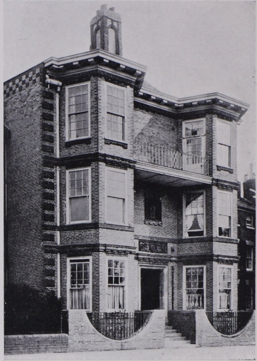
QUEEN'S COURT, HAGLEY ROAD, BIRMINGHAM. THESE FLATS ARE THE FIRST WHICH HAVE BEEN BUILT IN BIRMINGHAM, AND THEIR RENTS VARY FROM £80 TO £100 PER ANNUM. THE PLAN SHOWS THE TREATMENT OF A LONG AND VERY NARROW SITE, WITH THE CENTRAL ROOMS LIGHTED AND VENTILATED FROM AREAS. THE ARCHITECT HAS MADE AN EXTENSIVE USE OF LUXFER PRISM GLASS, WHICH, FIXED AT CORRECT ANGLES, GREATLY INCREASES THE VALUE OF TRANSMITTED LIGHT, WHILE ACTING AS A SCREEN THROUGH WHICH TENANTS CANNOT SEE. THE LONG PASSAGES, UNAVOIDABLE IN NARROW SITES, HAVE THE GREAT ADVANTAGE OF BEING WIDER THAN IS USUAL IN FLATS, THEIR WIDTH RANGING FROM THREE FT. TO THREE FT. NINE IN., AND FROM FOUR FT. TO FIVE FT. THREE IN. TWO FLATS ON THE GROUND FLOOR ARE REPRESENTED IN THE PLAN
