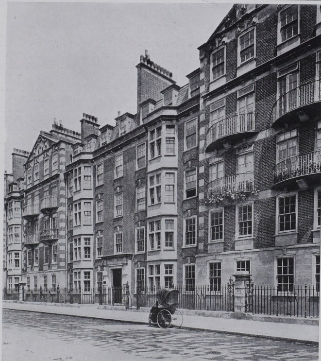
COLEHERNE COURT, OLD BROMPTON ROAD, LONDON. AN EXAMPLE OF EXTERIOR DESIGN, WITH PLEASANT WINDOWS OF A KIND NOT COMMON IN FLATS. THE BUILDING MATERIALS ARE RED BRICK WITH BATH AND PORTLAND STONE. THE RENTS, INCLUDING RATES AND TAXES, RUN FROM £140 TO £160 A YEAR
