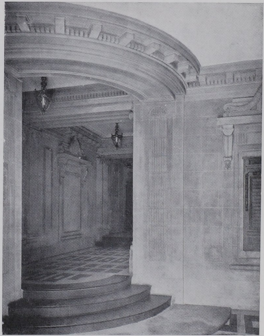
THE WORK IS CARRIED OUT IN STONE COMPOSITION NEAR THE ENTRANCE HALL
