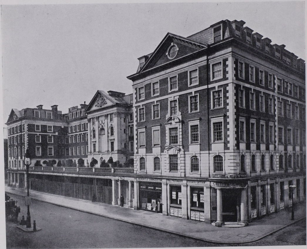
HORTON COURT, KENSINGTON, LONDON. SECOND FLOOR PLAN AND THE FRONT TO KENSINGTON HIGH STREET. THE MATERIALS ARE ENGLISH RED BRICKS, PALOTTE STONE FROM FRANCE, WITH PORTLAND STONE FOR THE GROUND FLOOR. THE SUITES OF ROOMS ARE DESIGNED FOR DIFFERENT INCOMES, SOME BEING SMALL AND OTHERS LARGER. THE RENTS, INCLUDING RATES AND TAXES, RUN FROM £90 TO £210 PER ANNUM. NOTE THE GARDEN TERRACE ABOVE THE SHOPS, THE ABSENCE OF AN AREA, AND THE DIRECT WINDOW-VENTILATION GIVEN TO EACH CORRIDOR
