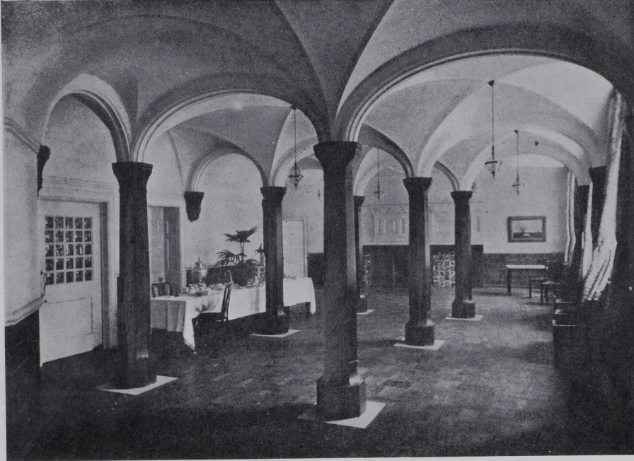
CAMPDEN HOUSE CHAMBERS, CAMPDEN HILL, KENSINGTON, LONDON. VIEW OF THE DINING-HALL IN A BLOCK OF CATERING FLATS. THE VAULTING IS CARRIED ON BLACK GRANITE COLUMNS; THE PAVEMENT IS OF TEAK
