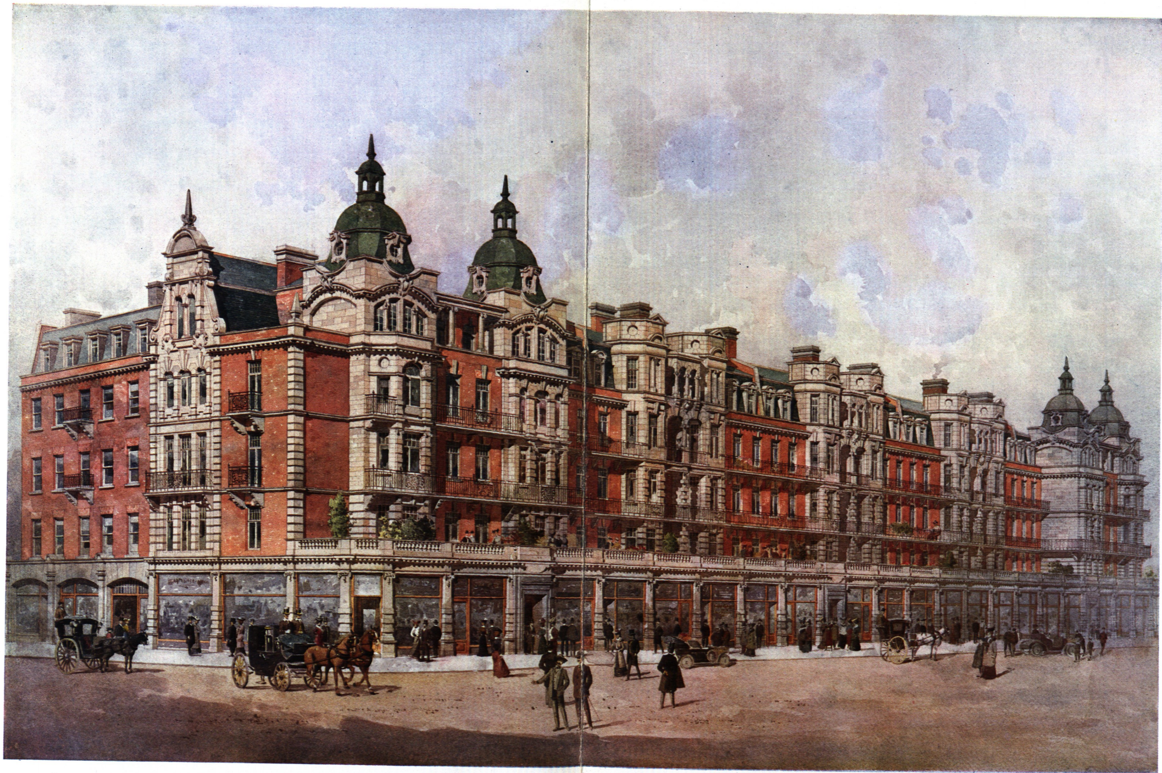
BLOCK OF FLATS, ST. GEORGE'S TERRACE, GLOUCESTER ROAD, LONDON, SHOWING THE ELEVATION WITH THE RETURN FRONTAGE TO ST. GEORGE'S PLACE, AND THE ROOF GARDENS ON THE FIRST FLOOR LEVEL.
