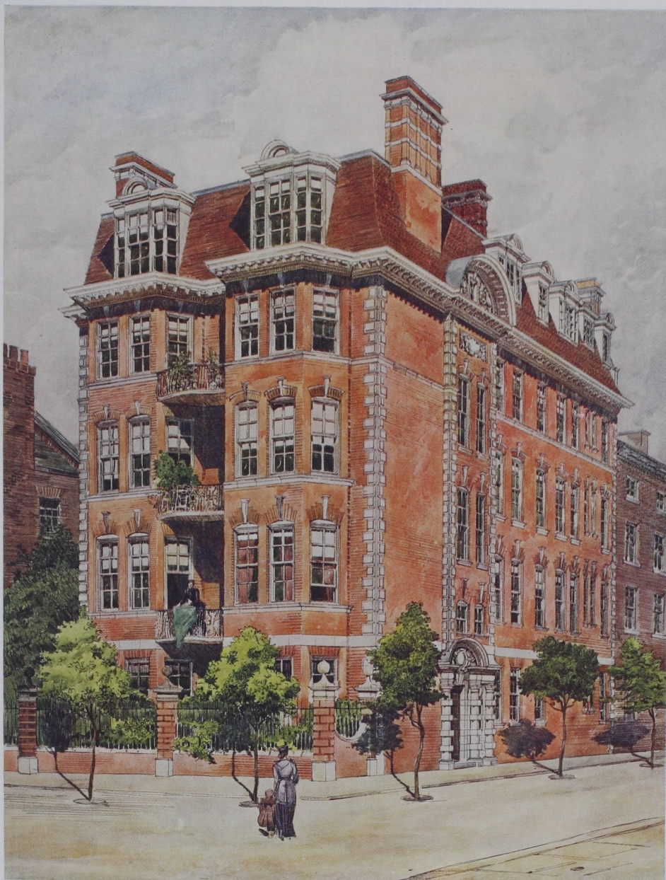
BLOCK OF FLATS, EARL'S COURT SQUARE, LONDON. MATERIALS: RED FACING BRICKS, BATH STONE DRESSINGS; THE ROOF COVERED WITH TILES, THE WOODWORK PAINTED WHITE
