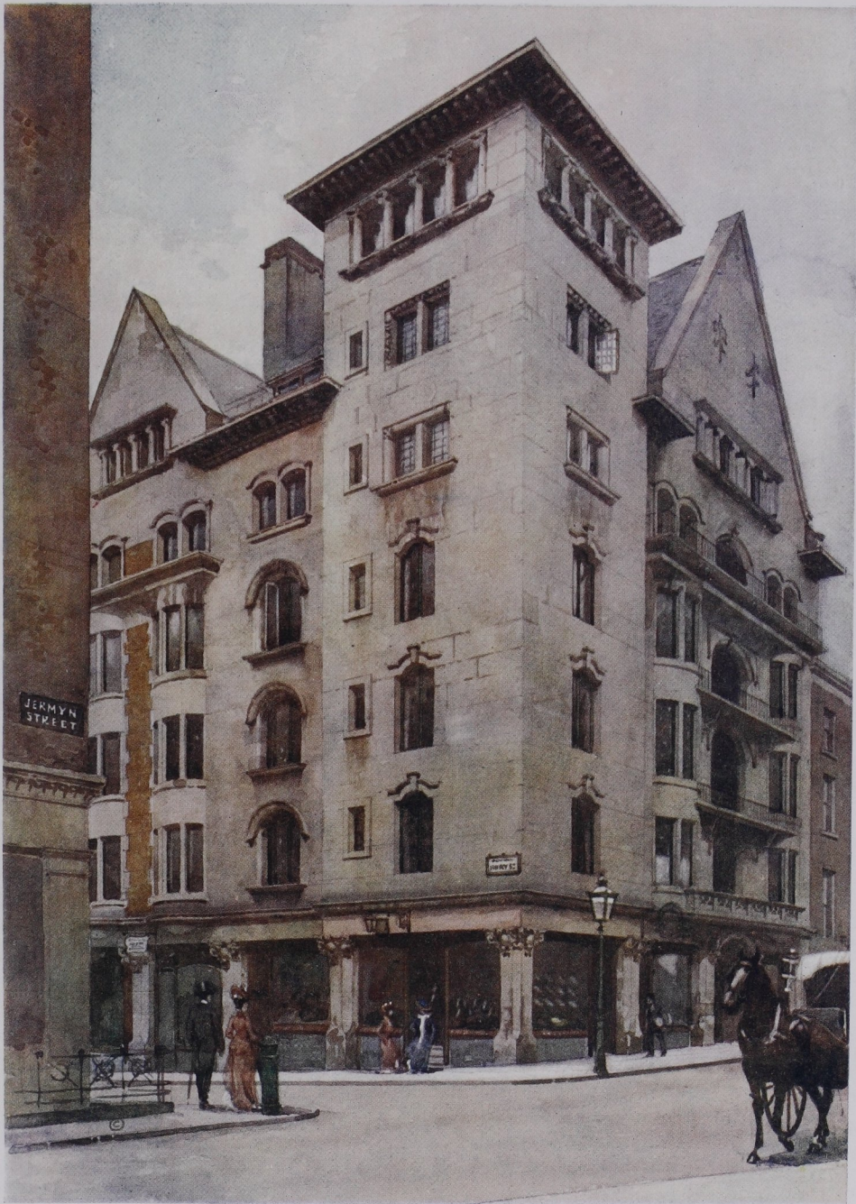
MARLBOROUGH CHAMBERS, JERMYN STREET, LONDON, W. FROM A DRAWING BY T. HAMILTON CRAWFORD. THE BUILDING IS FACED WITH PORTLAND STONE AND BACKED WITH BRICKS. THE HEIGHT FROM THE GROUND FLOOR TO THE TOP STOREY IS 54 FEET; FROM THE GROUND LEVEL TO THE CORNER OF THE TURRET, 74 FEET; AND TO THE TOP OF THE GABLE, 86 FEET
