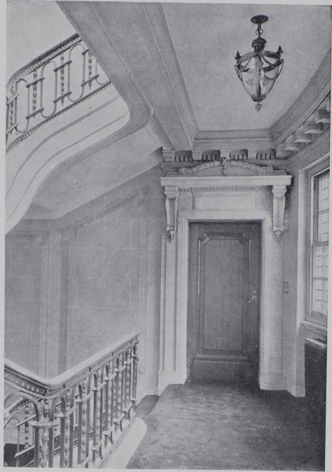
THE WORK IS CARRIED OUT IN STONE COMPOSITION ON THE STAIRCASE
