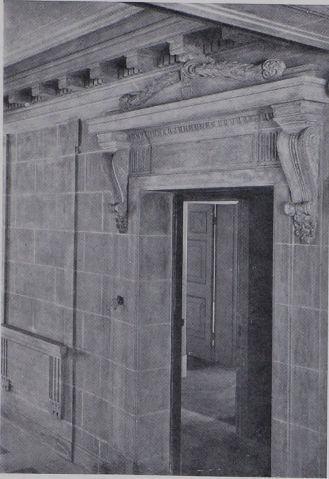
MANSION FLATS, 25, BERKELEY SQUARE, LONDON ON THE GROUND FLOOR
