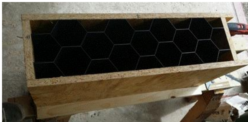
Figure 3-2: Shuttering for hexagonal shaped fillings.
