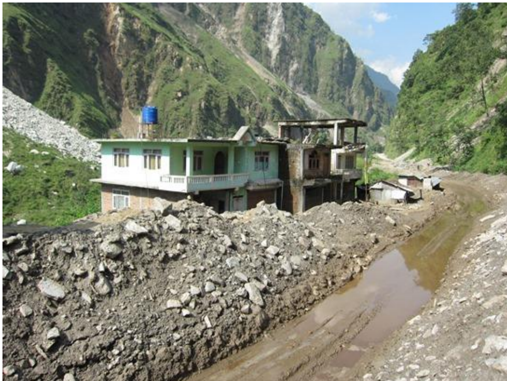
Figure 67 Massive debris masses blocked the roads during and after the monsoon (© Ziselsberger) 27°54'23.37"N, 85°55'15.37"E
