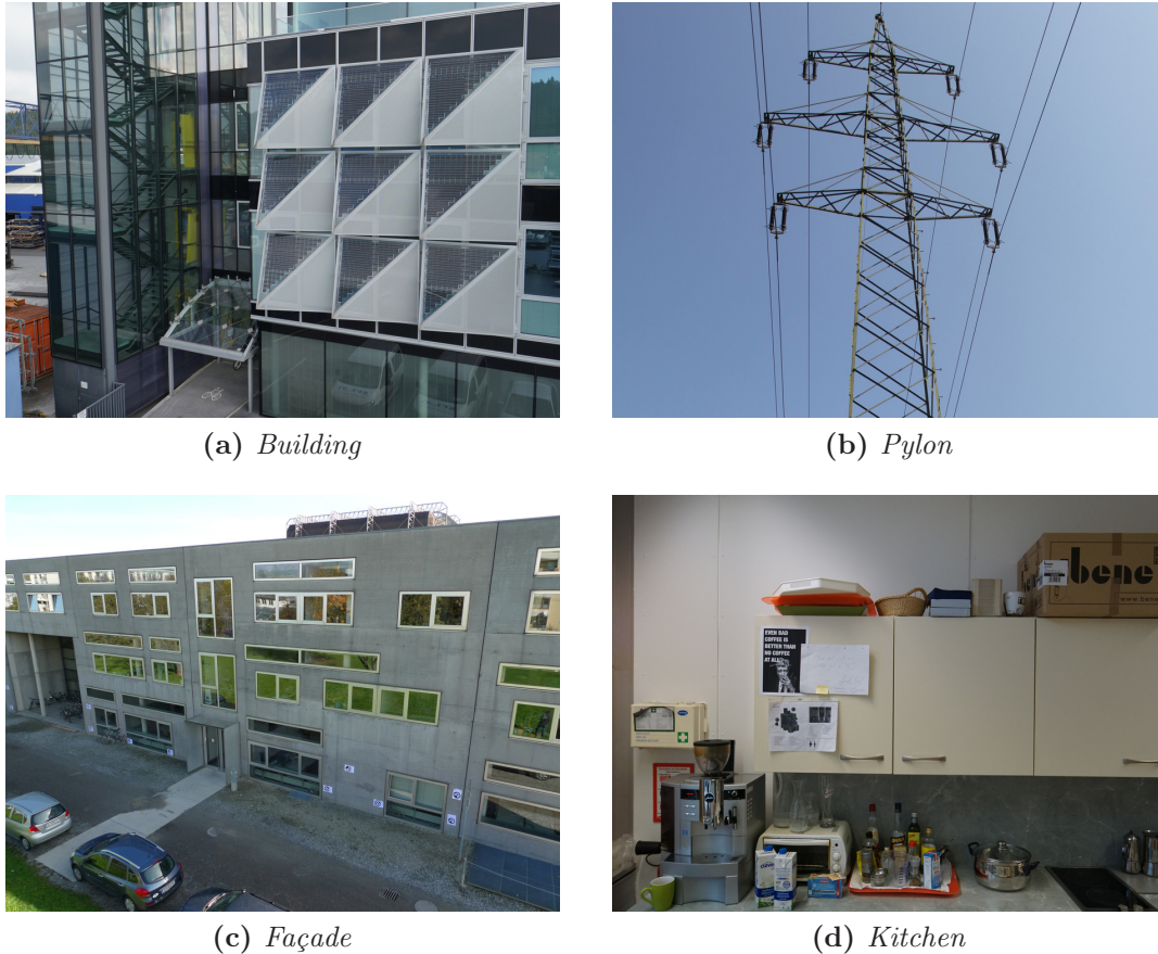
Figure 4.3: Example images from the real-world sequences (a) Building , (b) Pylon , (c) Façade , and (d) Kitchen . Information about the datasets can be found in Table 4.2.
