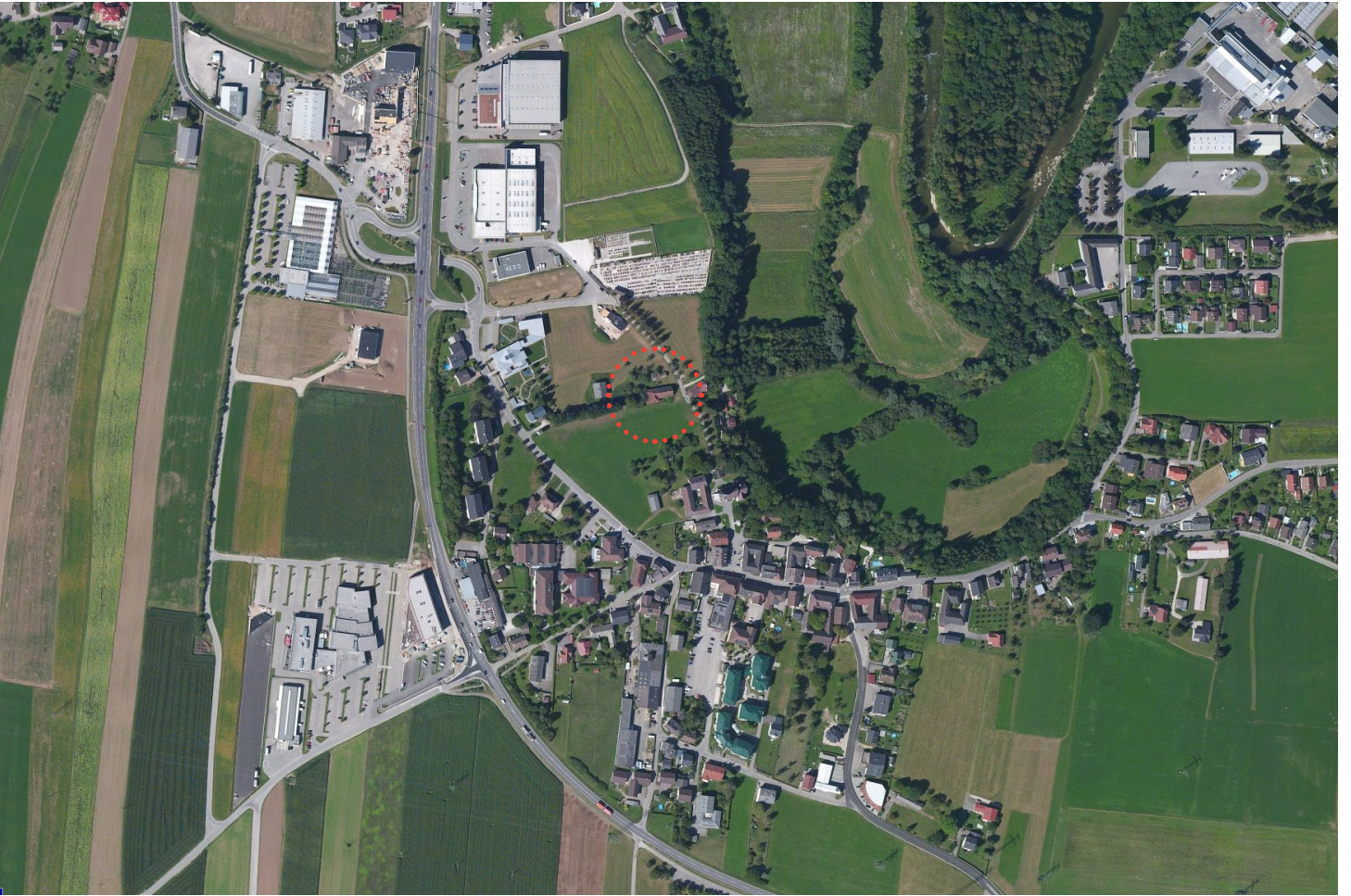
AERIAL VIEW OF THE BUILDING SITE
