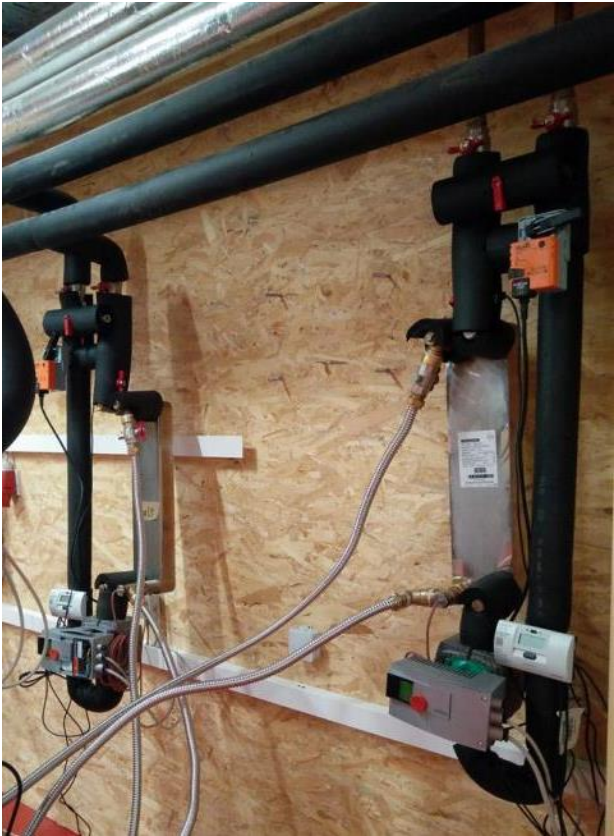
Figure 66: Hot and cold water circuit, on the right side connected to the test rig, on the left side connected to the labor
