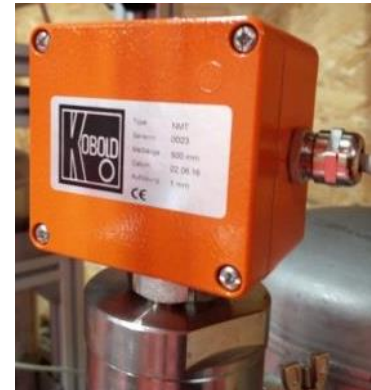
Figure 27: Head of the liquid level measurement
