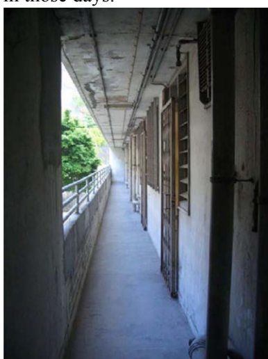
Abb. 147: View of Corridor
