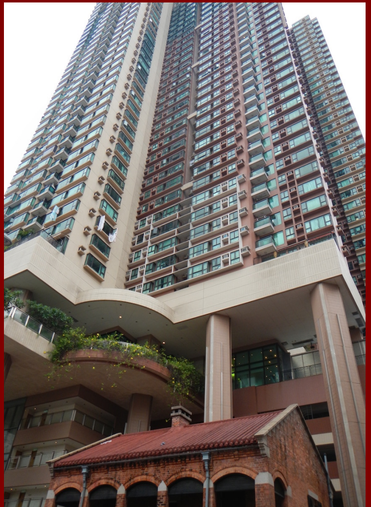
Abb. 181: Modern Resettlement Block
