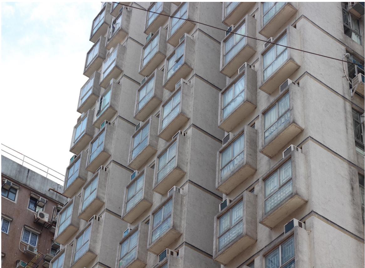
Abb. 260: Huge Glass Surfaces makes difficult for a comfortable well-being inside the flats of Hong Kong Island
