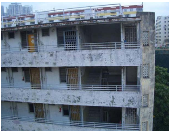
Abb. 152: Veranda at the Upper Floors
