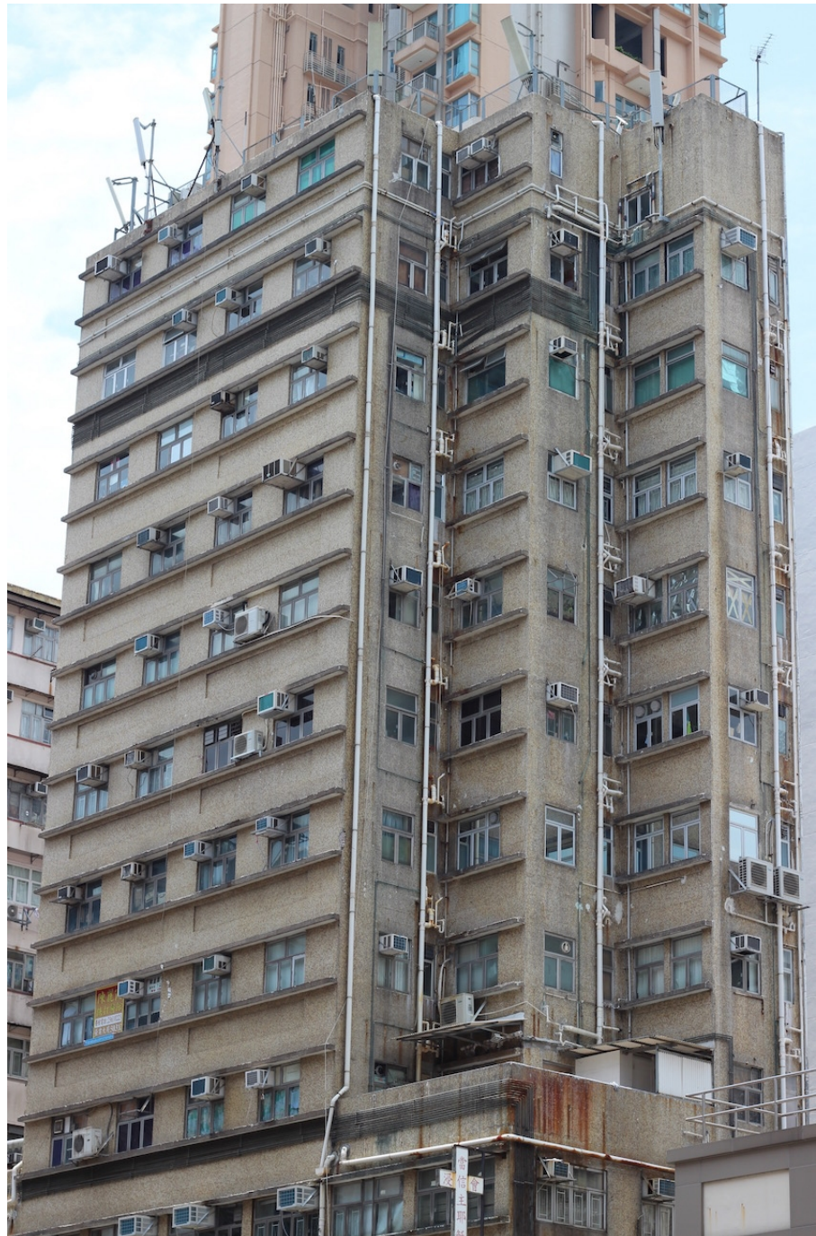
Abb. 267: Pipes and Wires are always on the Facade of the older Buildings to save Space inside
