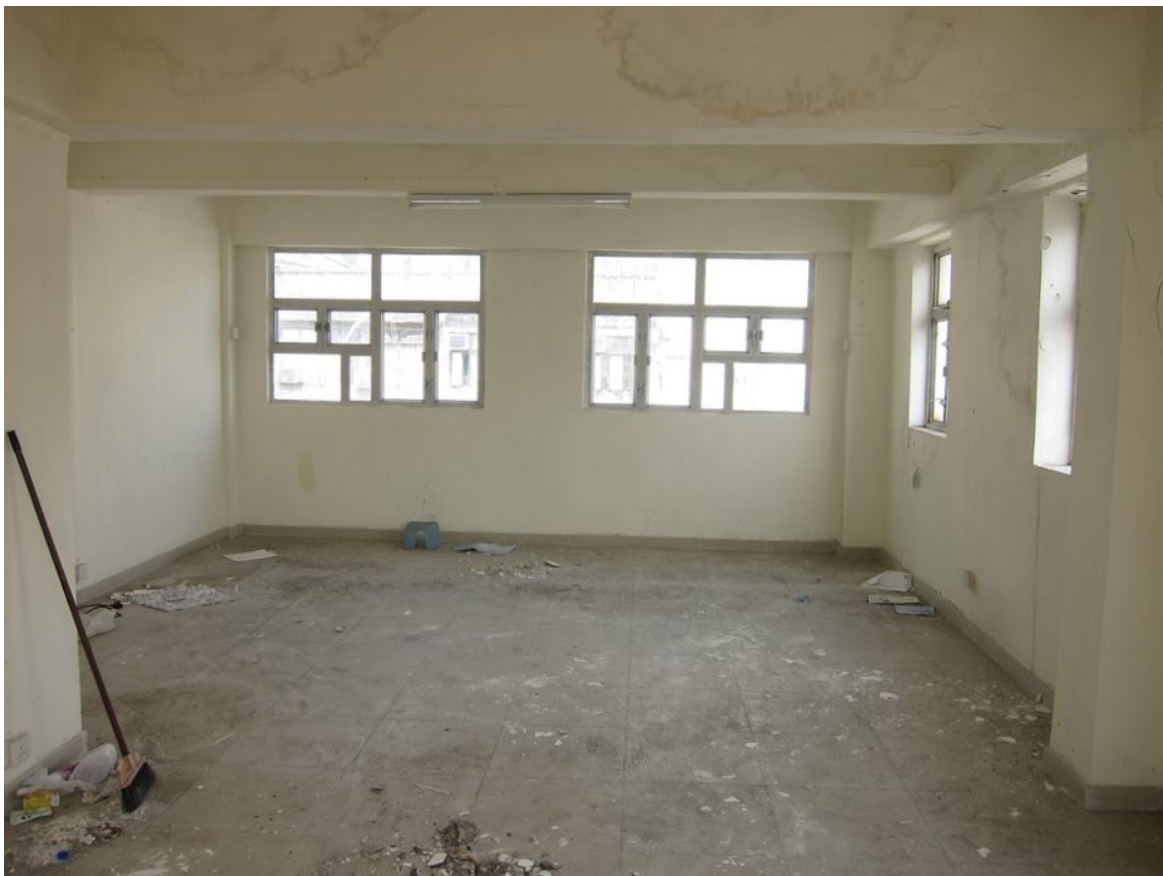
Abb. 253: The Apartment during renovation around 2010
