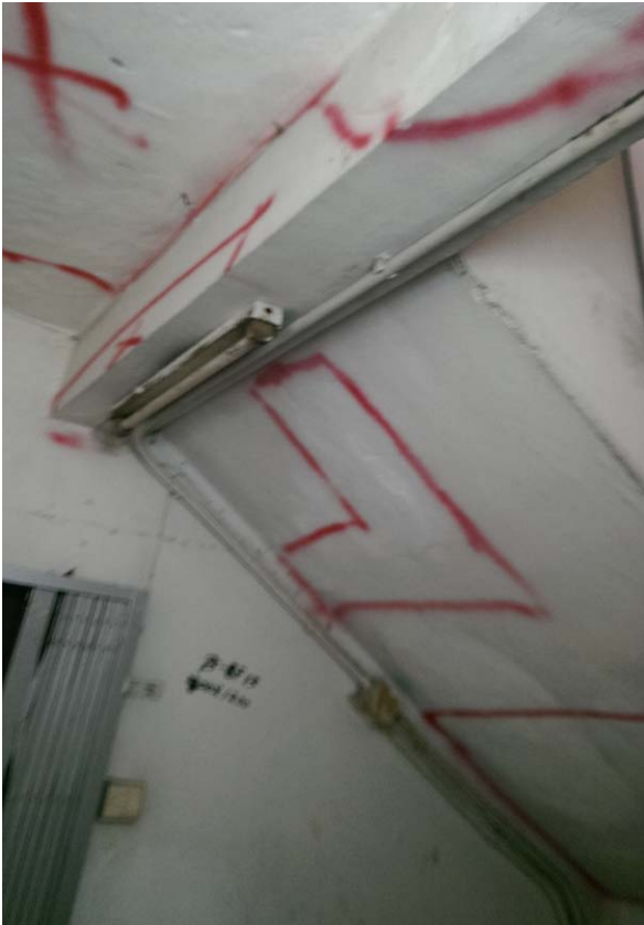
Abb. 265: Damages due to damp were marked in the Staircase of my Apartment
