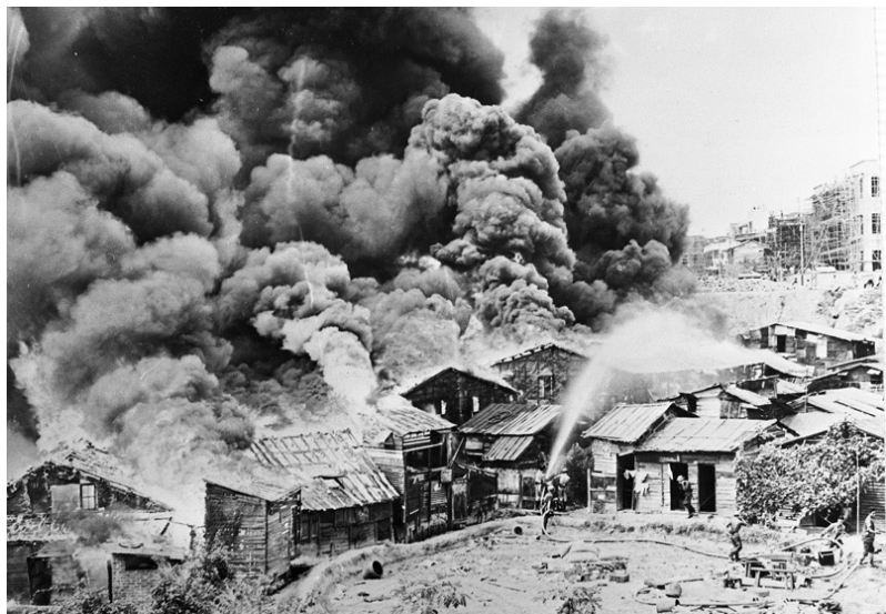
Abb. 81: Fire Brigade tries to extinguish fire
