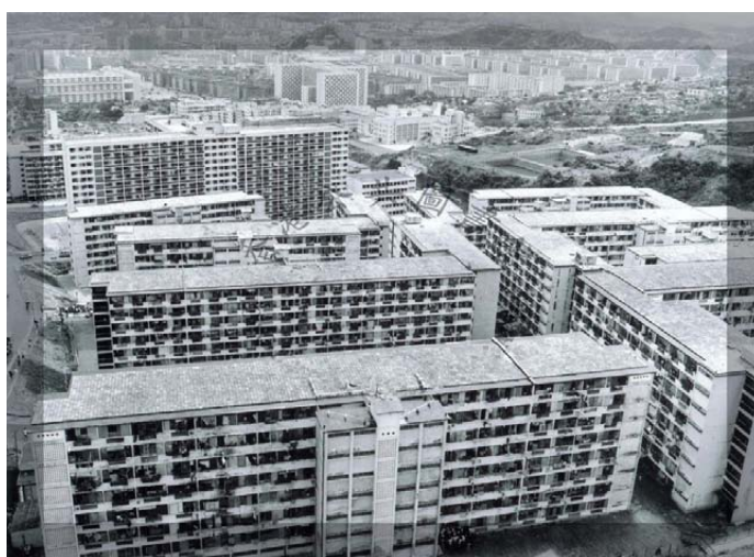
Abb. 117: Tsz Wan Shan Resettlement Blocks
