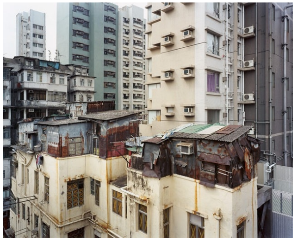
Abb. 67: Illegal Corrugated Metal Roof Houses
