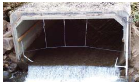
Abbildung C 1-9: CIRCULAR Antenne (Düker) (Oregon, 2009)
