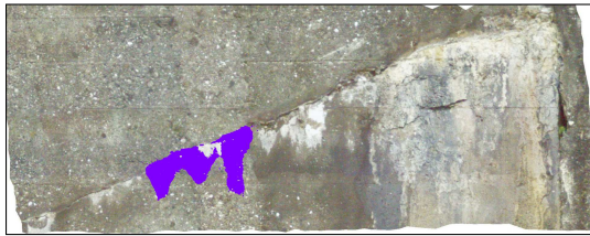
(a) Identified changes by applying DBSCAN algorithm to the segmented difference image I_b
