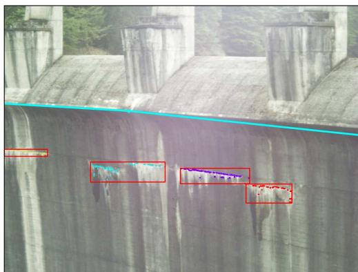
(a) Illustration of MBR (red rectangles) of detected defects after filtering; cyan line represents the outline of the filtering polygon
