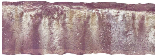
Figure 5-10: Exemplary orthophoto of a defect with ambiguous crack path
