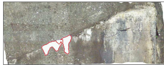
(b) Identified changes by finding their contours in the binary image I_b
