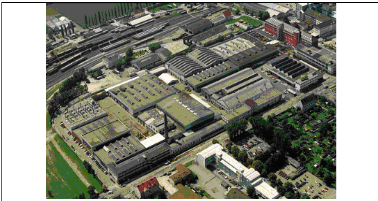
Figure 12: Siemens Plant in Graz, Eggenberg Source: Siemens internal presentation (2010)
