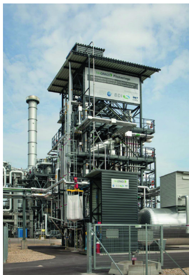
Fig. 1 bioCRACK pilot plant at OMV refinery Vienna/Schwechat.
