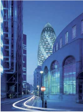
FIG. 77 The SwissRe high-rise building in London is a new landmark of London's skyline.
