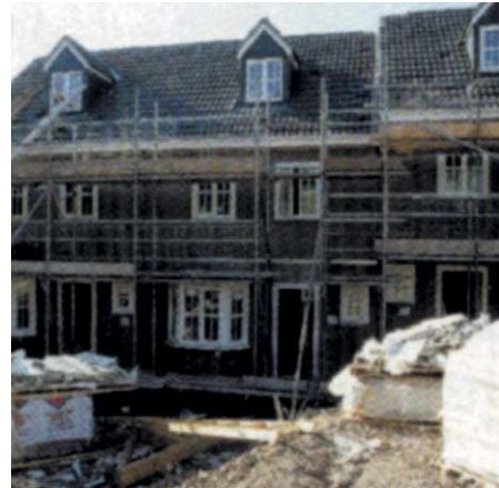
FIG. 97 The factory-made houses are not distinguishable from the traditionally built home. (source: www.space4.com ).
