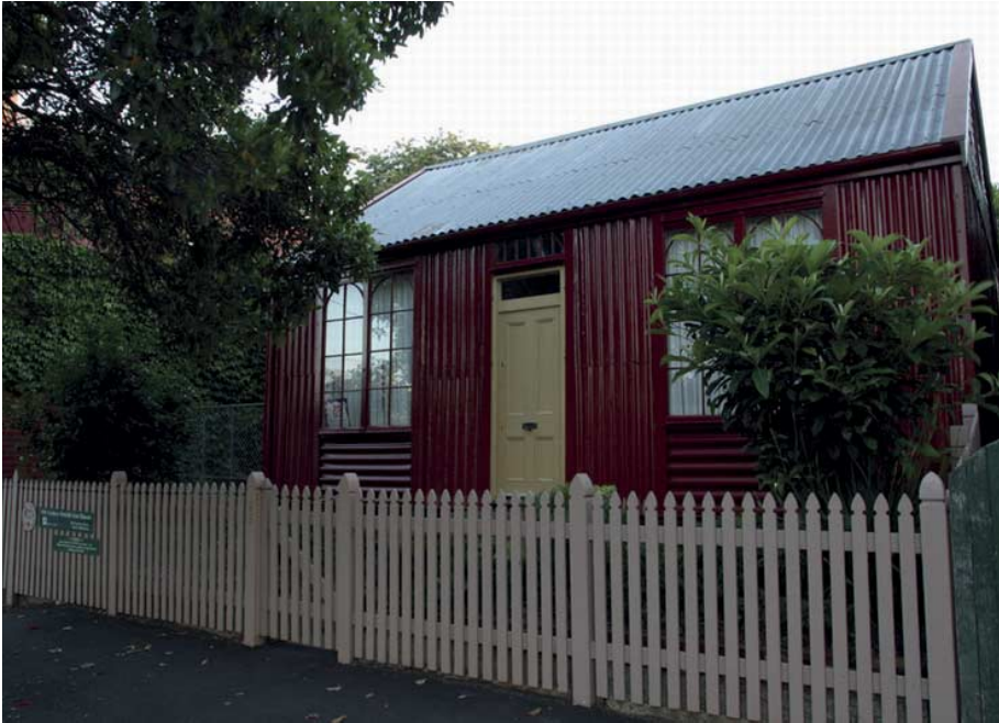
FIG. 06 The Portable Iron House was imported and erected in 1853-54 for local speculator Robert Patterson is still located on the original site, fronting 399 Coventry Street South Melbourne. The portable iron structure, of utilitarian design and unknown manufacture, is constructed of a tee and angle section wrought iron frame clad with five inch pitch corrugated sheet, which is partitioned and lined internally with horizontal boards to form an attic cottage of six rooms. [Source: www.onlymelbourne.com.au ]
