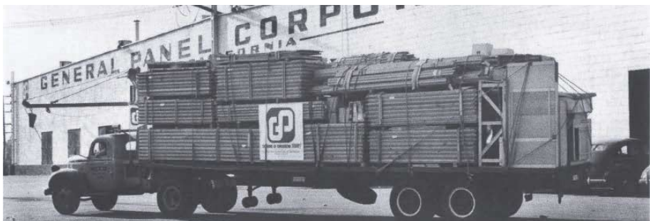
FIG. 19 General Panel, California, components being shipped by truck from factory, c. 1947 [source: Ludwig, 1998]
