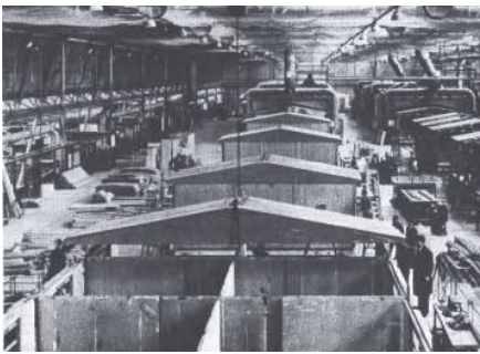
FIG. 25 Aluminium Bungalow, assembly line production, 1947 [source: Herbert, 1984]
