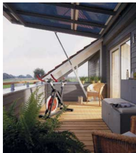
FIG. 82 The 'Cabrio-Haus' offers a glazed roof section, which can be opened like in a convertible car. (source: www.baufritz.com )
