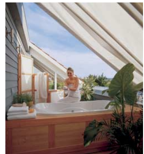
FIG. 82 The 'Cabrio-Haus' offers a glazed roof section, which can be opened like in a convertible car. (source: www.baufritz.com )
