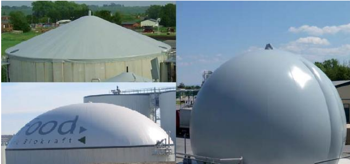
Figure 3: Different shapes of biogas storage tanks made by Sattler AG, conical (top left), \frac{1}{4} sphere (bottom left) and \frac{3}{4} sphere (right) (Sattler AG, 2012)
