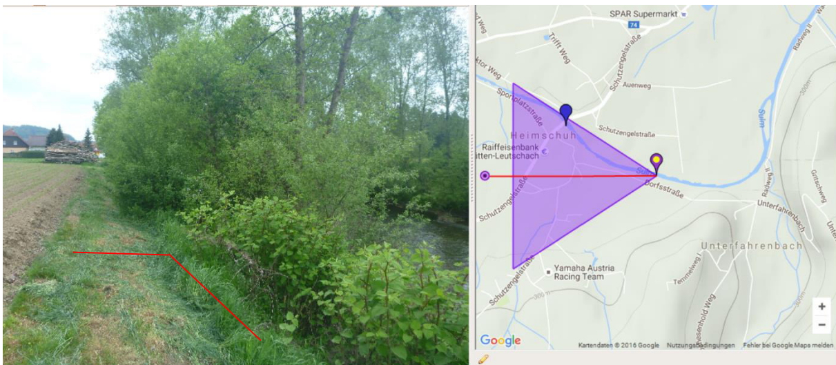
Figure 56 Steep bank between P120 and P119
