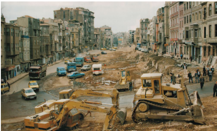
Figure 13. Construction of Tarlabası Boulevard, 1986.
