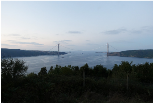
Figure 5. Unfinished Third Bridge, viewed from Beykoz, 2015
