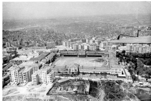
Figure 20. Aerial View of Taksim Square, before the demolition of the former Ottoman barracks
