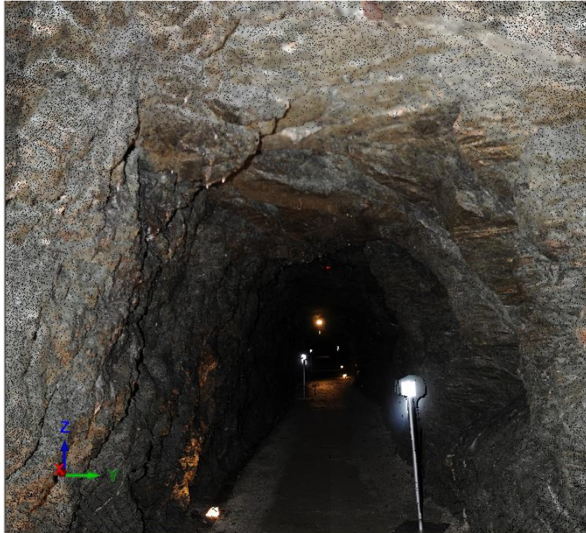
Figure 4.7: Screenshot of 3D LiDAR point cloud model: removed rock wedge right of reflector, view to the west (After Liu and Kieffer, 2012)
