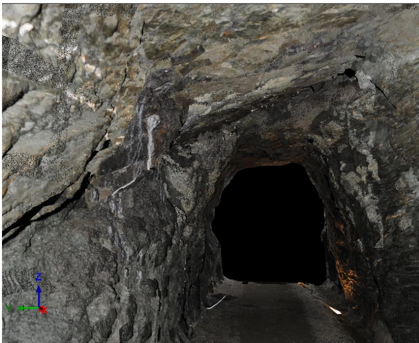
Figure 4.8: 3D textured mesh of fault zone, view to the east (After Liu and Kieffer, 2012)
