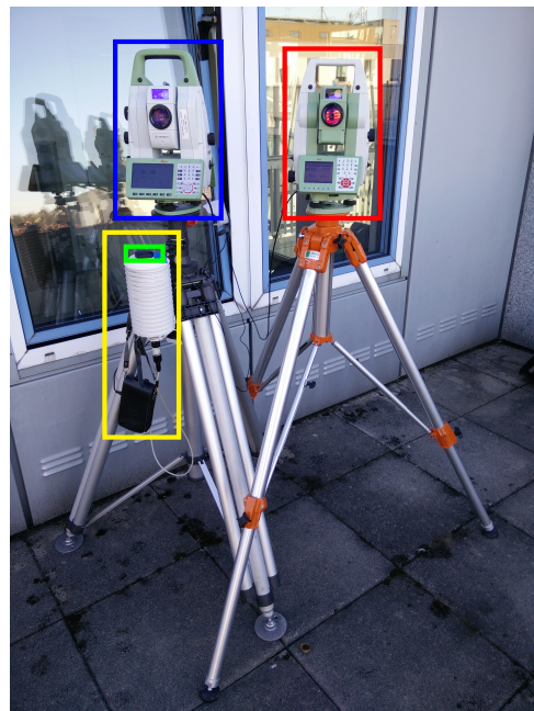
(b) Outside the building (green - GPS antenna, blue - Leica MS60, red - Leica TS15, yellow - weather station)
