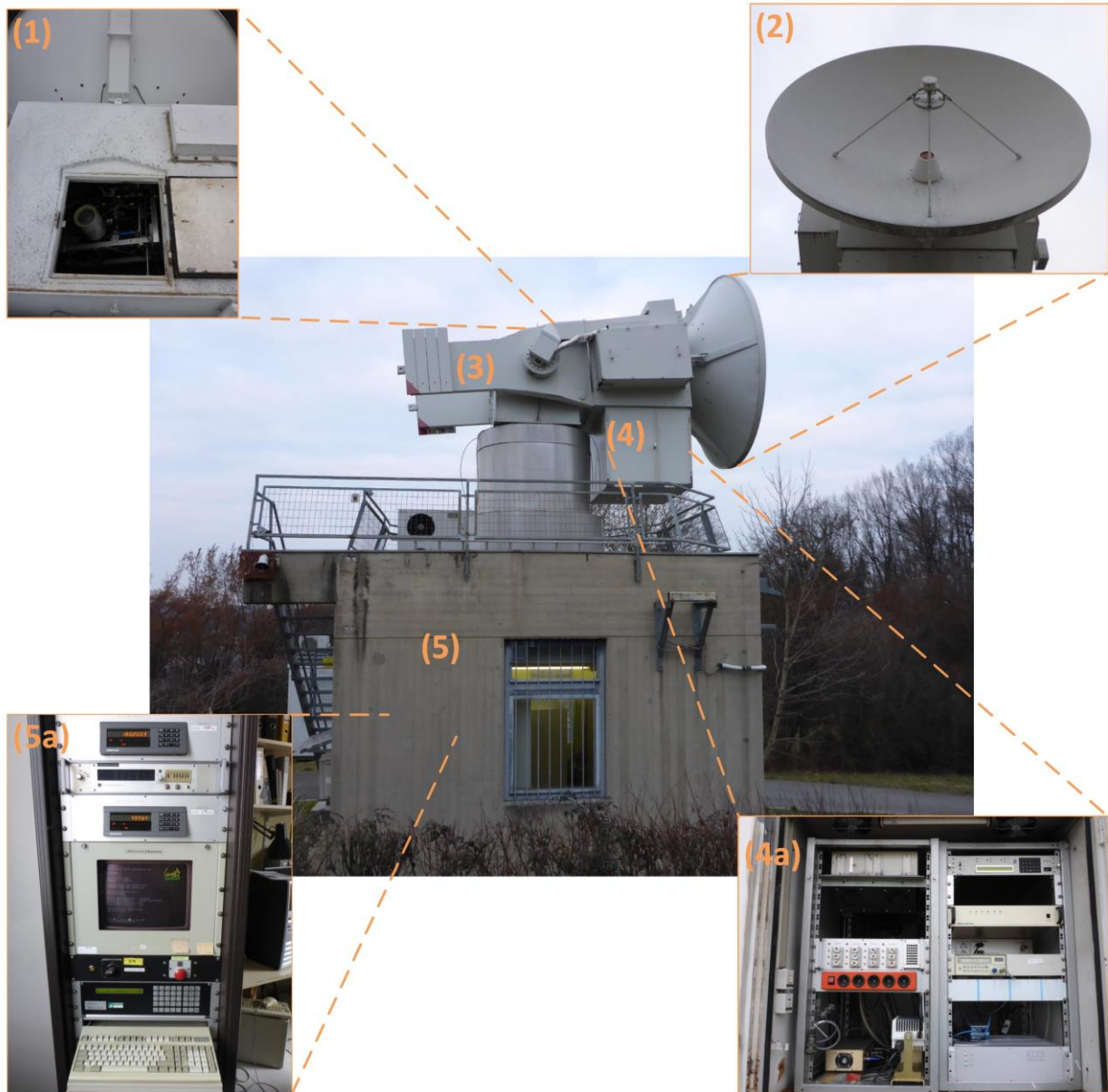
Figure 2-1 Ground station building of the Lustübhel satellite station. (1) Shows the open hatch on top of the antenna pedestal, providing access to the waveguide housing. (2) Antenna and Cassegrain feed. (3) Antenna pedestal, holding the antenna and the antenna hardware box. (4) Antenna hardware box that provides space for hardware and cables. (5) Ground station building. (5a) Ground station control rack.
