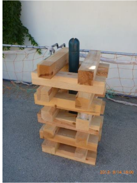
Figure 1.2: Example shoring task [5]
