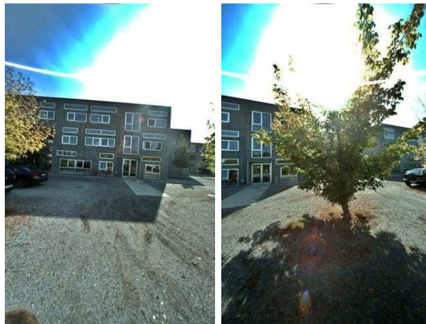
Figure 5.12: Left: Excerpt from the texturing result of dataset 1 (Inffeldgasse). Below the two corresponding photos. The photo on the right has been used first for mapping. That's why the tree is on the building's texture even though on the left photo the view would have been clear (first-come first-serve principle of the texturing process).
