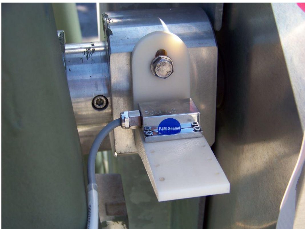
Figure 68: Adapter piece with PJM400/1 attached; mounted on the HVCB's shaft.
