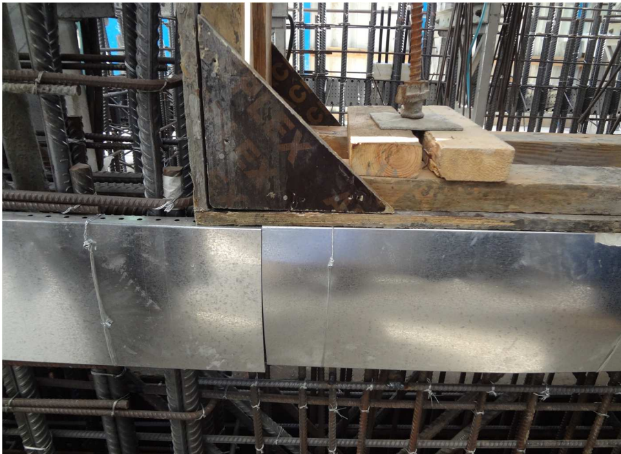
Fig. 4.11 Built-in part in metal, block-out in wood
