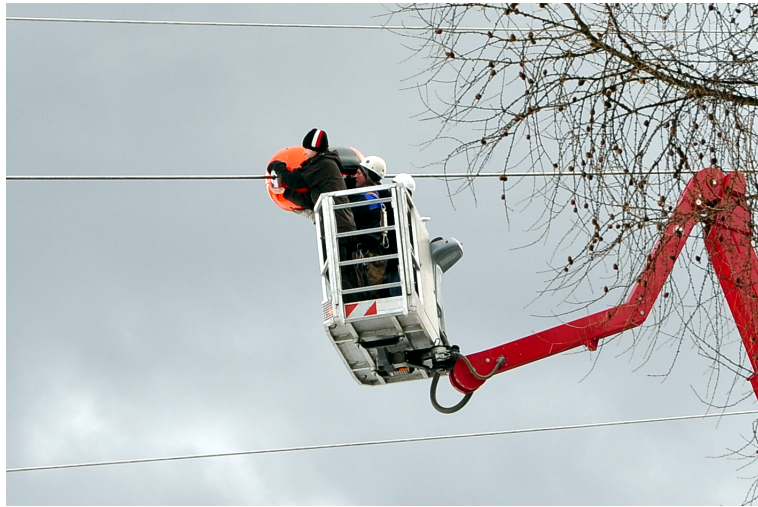
Figure 8.1: Mounting the test device onto the conductor rope, February 2010.
