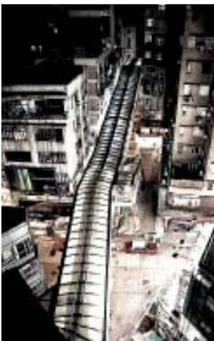
065 Structure from above
