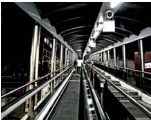
064 Inside the the Mid-Level Escalator
