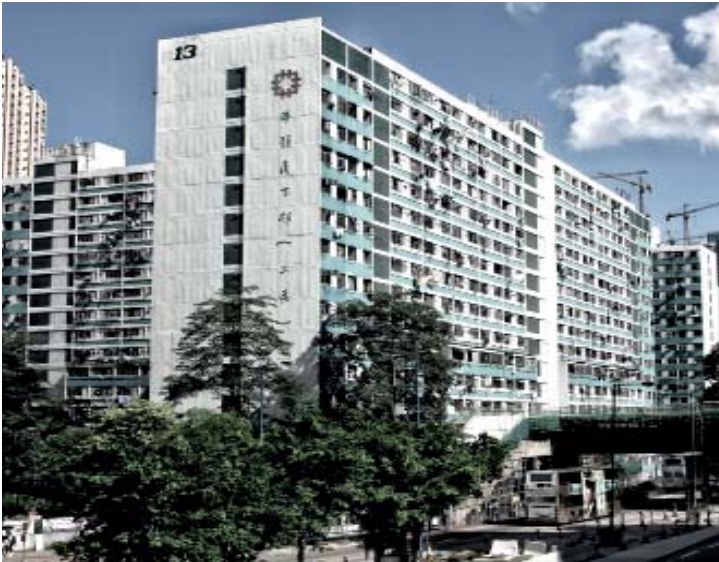
149 Lower Ngau Tau Kok Estate built 1969
