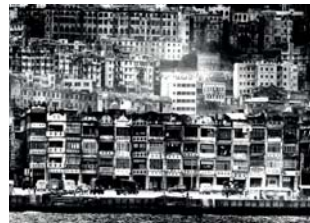
022 Connaught Road shop houses
