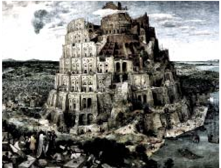
102 Construction of the Tower of Babel
