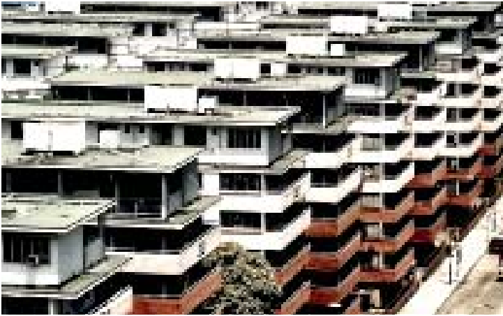
143 Shek Kip Mei resettlement Estate before demolition
