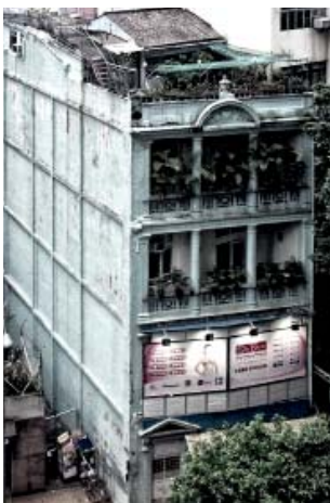
139 Shop house balcony type
