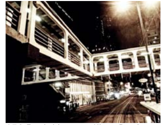
059 Footbridge over Kings Road
