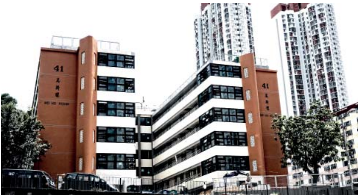
145 Refurbished Mei Ho House in 2013
