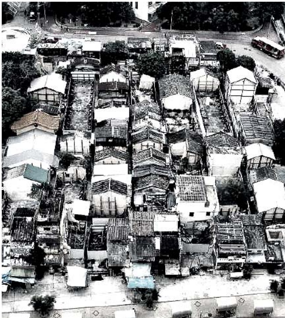
213 Nga Tsin Wai Village before demolition
