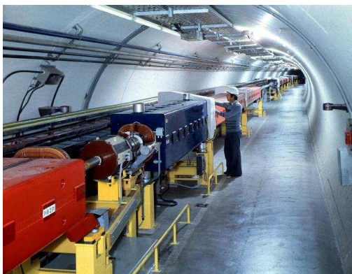
Figure 5.1: A view of the SPS tunnel.
