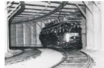
fig. 11 Tremont Street Subway
