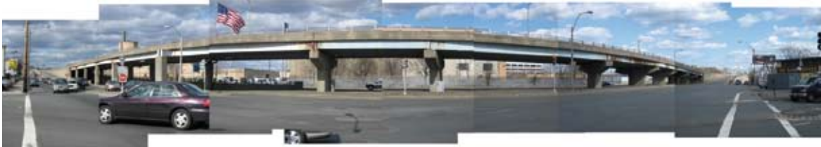
fig. 30 McGrath Highway at Somerville Avenue Intersection
