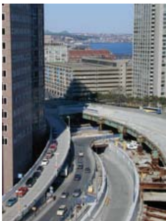
fig. 21 Building the Big Dig
