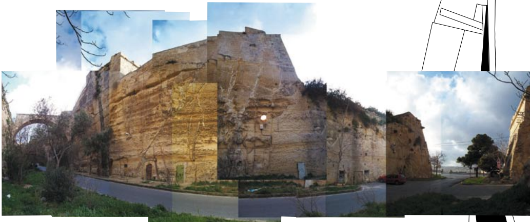
4.38 View 2. The doors of the shelters of WW2 are blocked up 100
