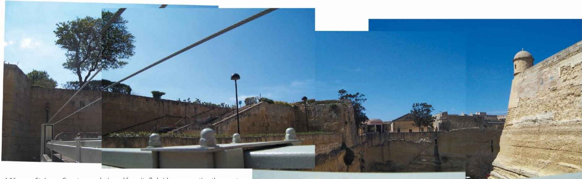
4.36 St. James Counterguard, viewed from its fly bridge, connecting the counter-guard with the bastion. The fly bridge was renovated and is used as an access for the National Bank's Garage underneath St. James Bastion
