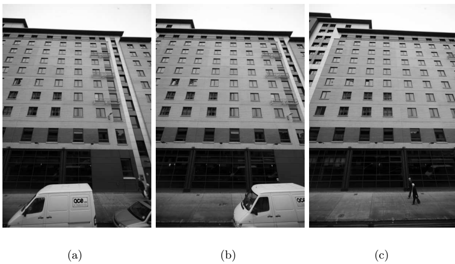
Figure 5.23: Three images of a modern facade with many repeating structures.
