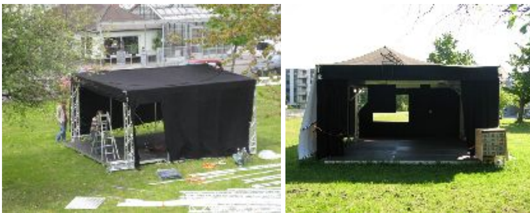
Figure 14: MR Tent Construction and First Assembly
