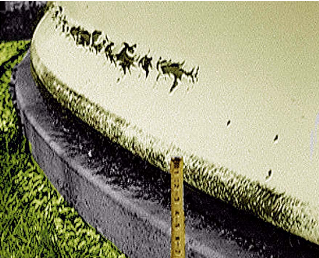
Figure 1.1 Elephant's foot buckling (JM Rotter)
