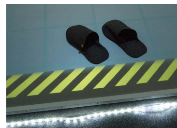
Figure 2.27: An LED strip is used to highlight the small step into the DAVE to avoid injuries. The floor projection is protected against dirt and scratches by felt slippers.
