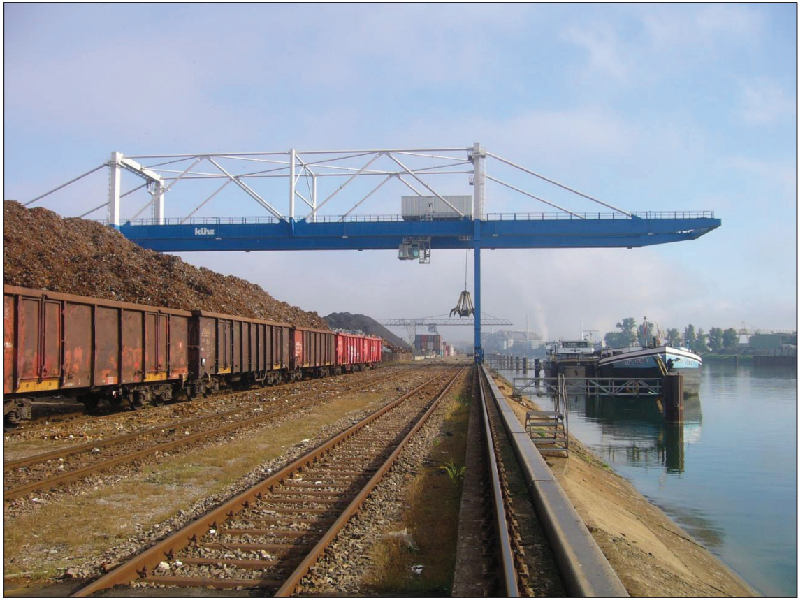
Figure 2-4 Kuenz RMG with an Attached Claw Fastener Instead of a Spreader 31
