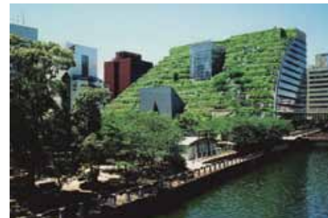
Abb. 24 Acros Building, Fukuoka, Ambasz
