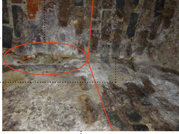
Abb 39 S3 Baufuge
