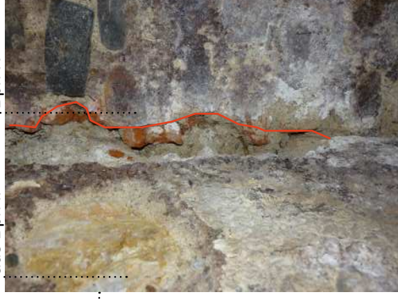
Abb 40 S3 Baufuge
