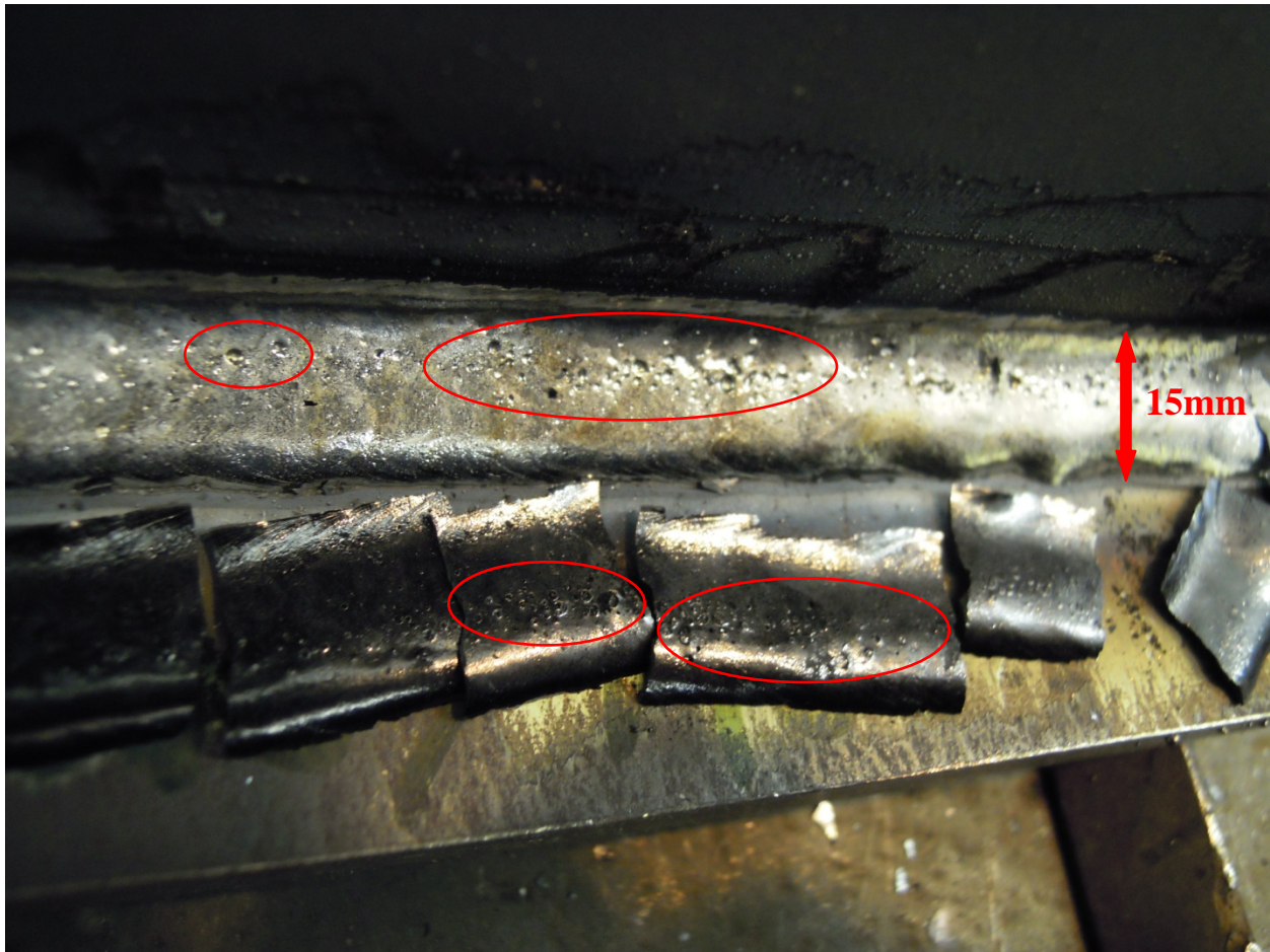
Figure 4-6: Dimples on a fillet weld (Masse 68)
