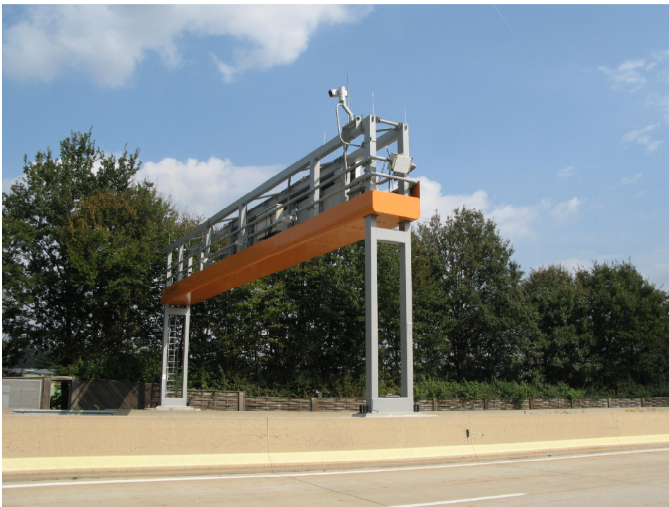
Figure 3: The picture illustrates the real system mounted on a highway gantry
