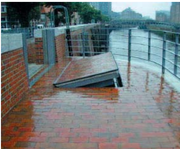
Abb. 75 Klappwand [86]
