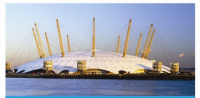
North Greenwich Arena 1
