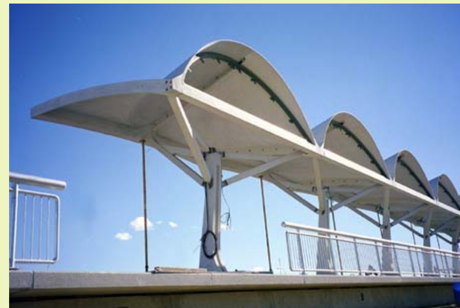
Abbildung 60: Shawnessy Light Rail Transit Station in Calgary/Canada
